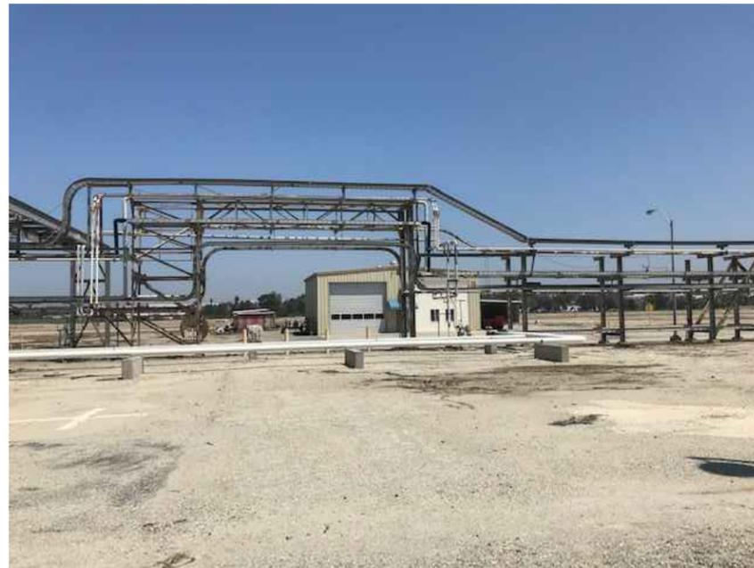
4) Existing east/west pipe rack that will convey the 4-inch natural gas line, view north
