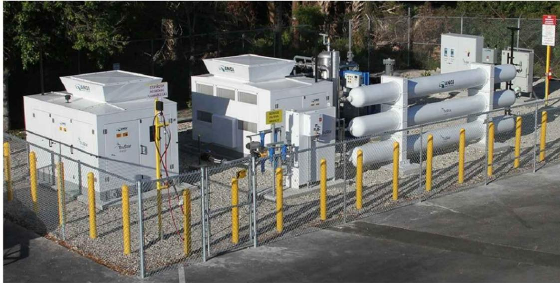
Typical CNG system compound, 2 compressors and 3 tanks
